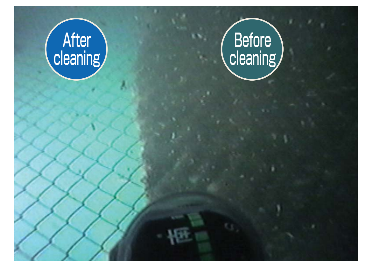
Video footage during cleaning of wire mesh net
